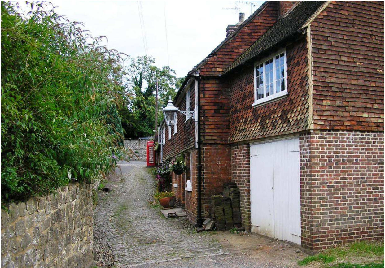
Historic cottages in Stairfoot Lane
