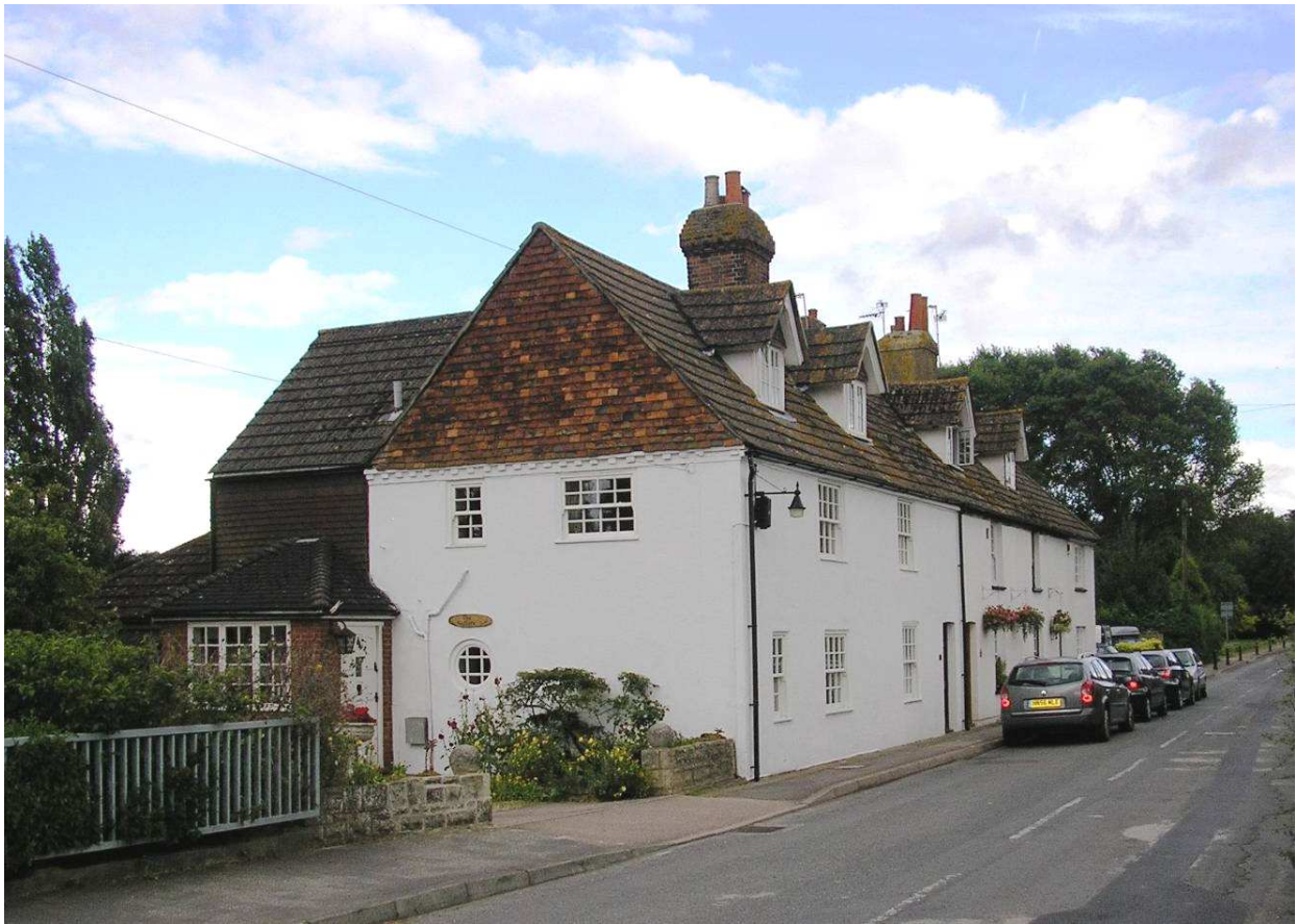
Historic cottages in Chevening Road
