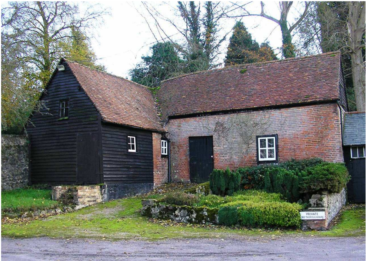
A limited palette of hand made vernacular materials adds to the character of this building.
