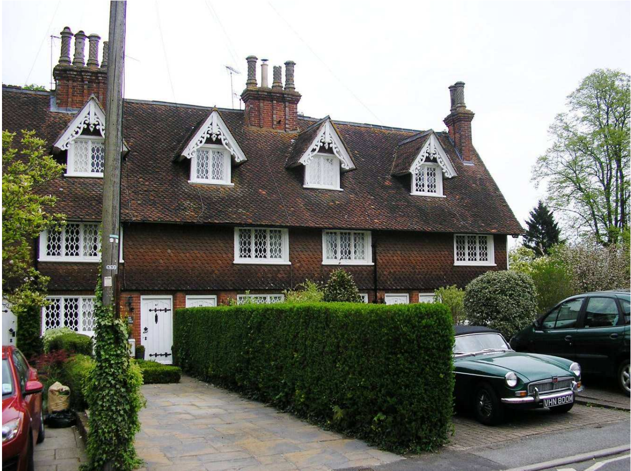
Former estate cottages, 43-53 High Street
