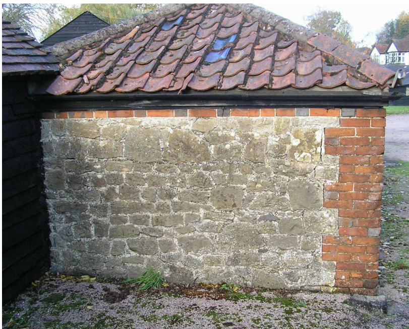
Simple vernacular detailing.
