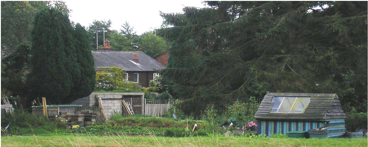
Locally distinctive allotment shed.
