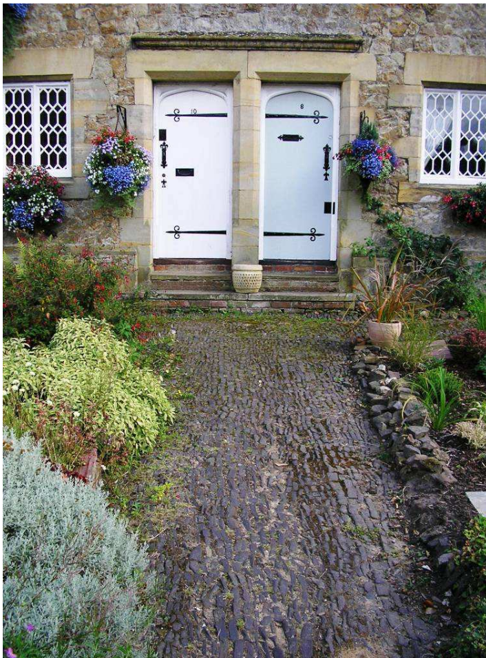
Locally distinctive details at the former Estate cottages
